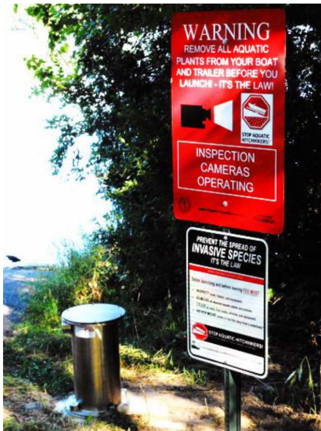
FIGURE 32. I-LIDS AIS SURVEILLANCE CAMERA SYSTEM
